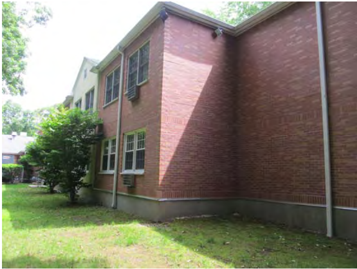
Typical panelized brick veneer exterior wall surface – No problems noted
