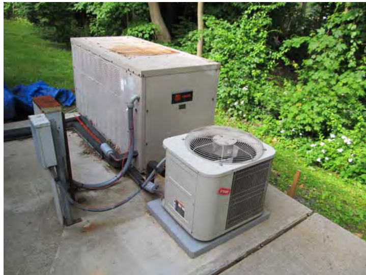
Exterior condenser units provide cooling capacity for select interior common areas
