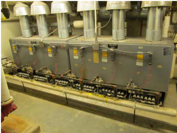
Original boiler plant serviceable but approaching the end of its expected useful service life
