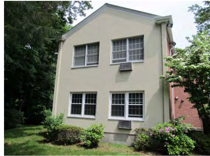
EIFS also used on some exterior wall surfaces
