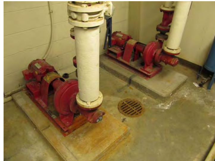
Base-mounted pumps for circulation of hydronic heat
