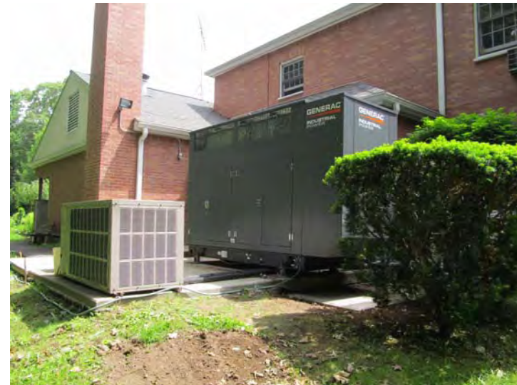
Recently installed (2013) emergency generator
