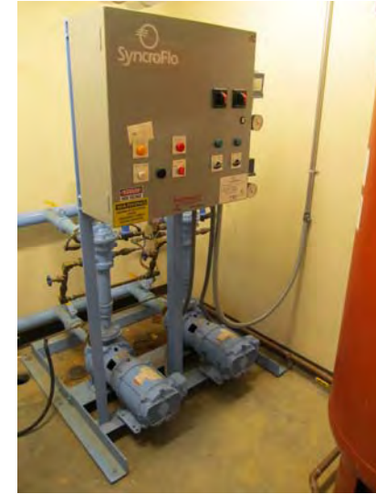
Duplex-type cold water booster pump station
