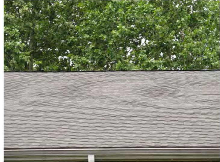
Architectural-type shingles on pitched roof surfaces are in good overall condition
