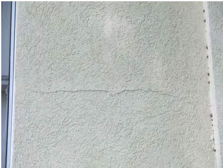
Age-related cracks noted in EIFS at isolated locations
