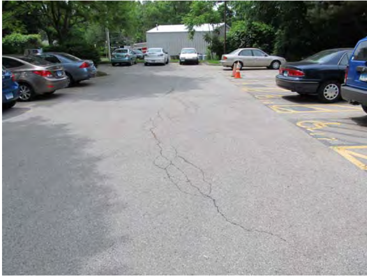
Asphalt paving in generally good condition – Surface maintenance needed in the near-term
