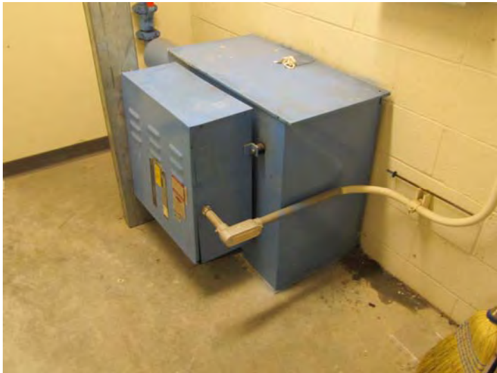
Hydro-mechanical pump station and controller/dispatcher unit for elevator
